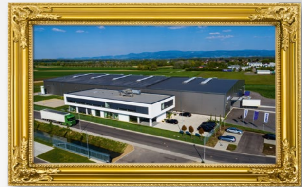
2017 New plant in Willstätt
